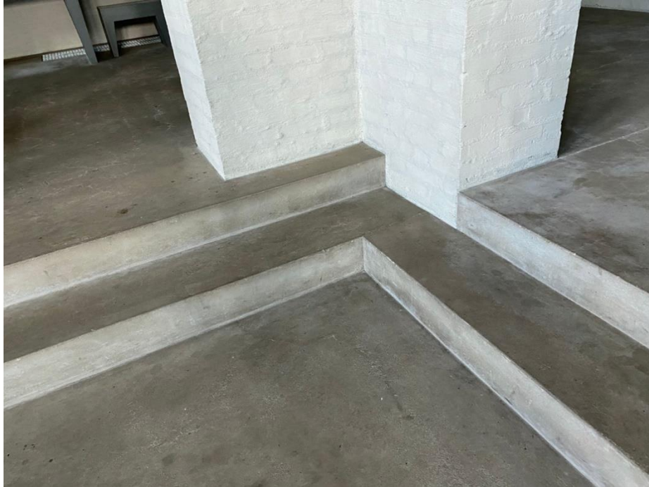
Figure 7: Detailing of the corner, column and steps. Photograph by author.
